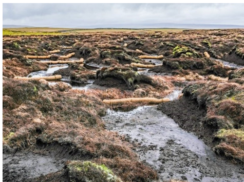
Coir logs are placed across eroded channels at Stake Moss to stop the peat washing away.
